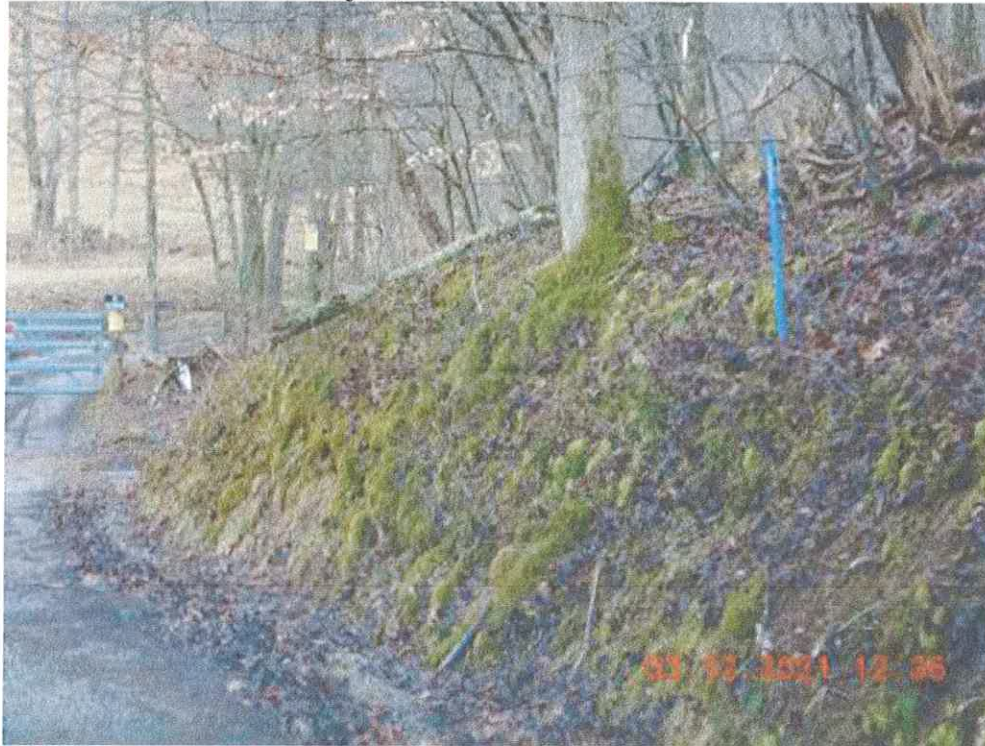
Site is stabilized and eligible for termination.
