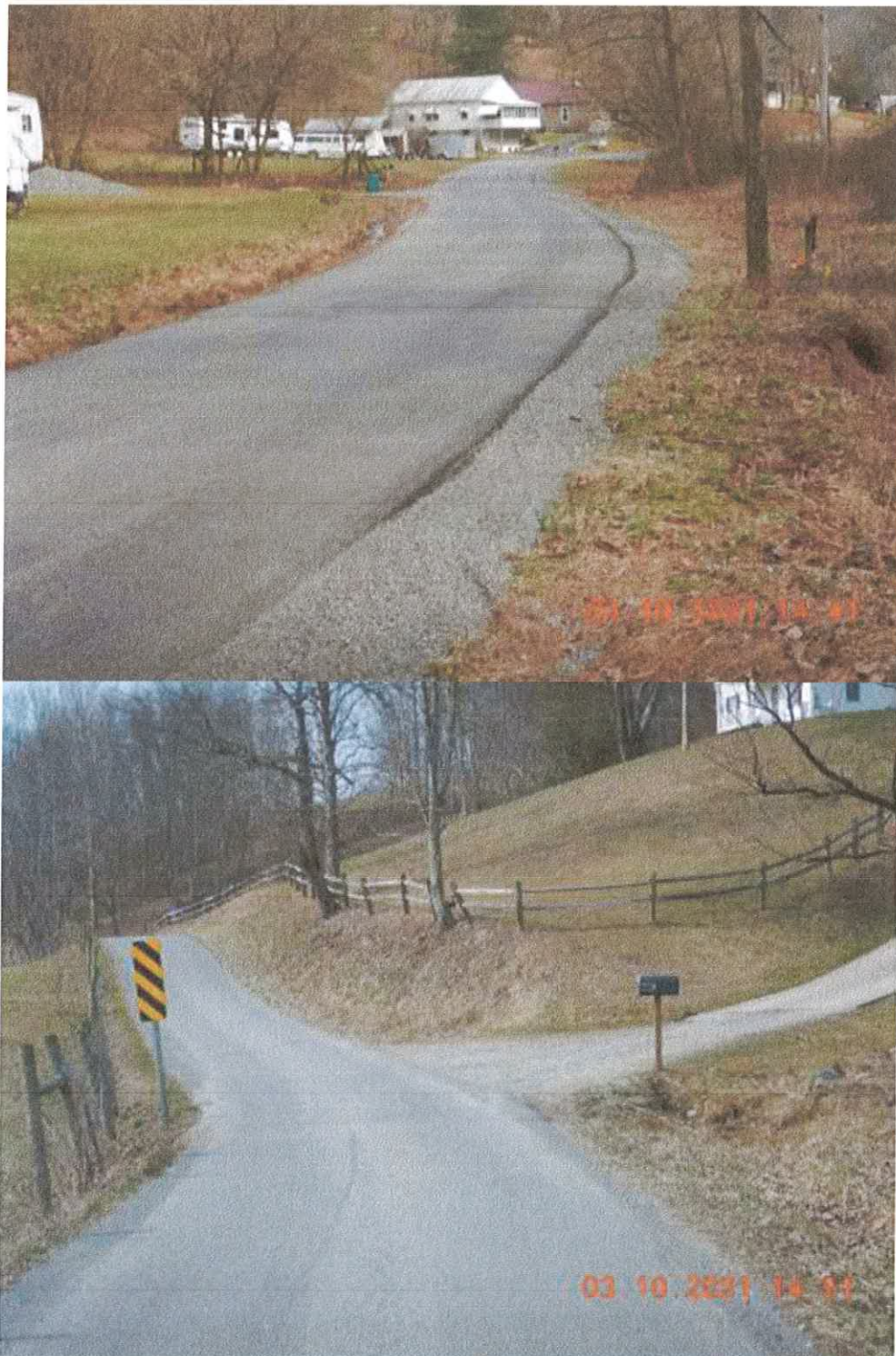
Site is stabilized and eligible for termination.
